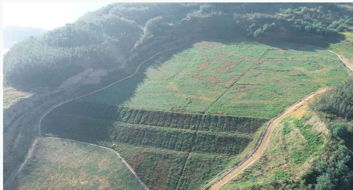
Ecological Restoration of Yunlong Phosphate Mine (After)
